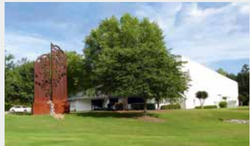
RAS Systems LLC in Georgia, USA
